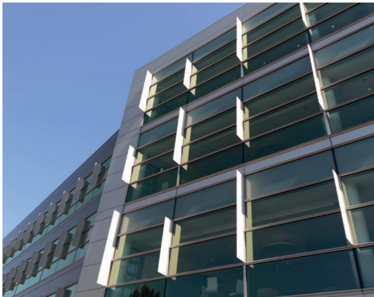
ABOVE: DuPont Chestnut Run building, Wilmington, Delaware, USA: Corian® Exteriors panels (made with Corian® Solid Surface Glacier White) were used to create sun shades offering a translucent glow during dusk and dawn, and also providing an interesting array of shadows across the building as the sun sweeps by throughout the day; project by AECOM; photo by Corian® Exteriors, all rights reserved.
